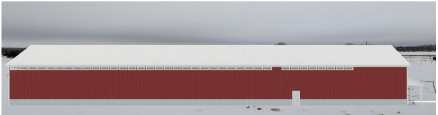
Backside of Building (opposite of Parking Lot)
