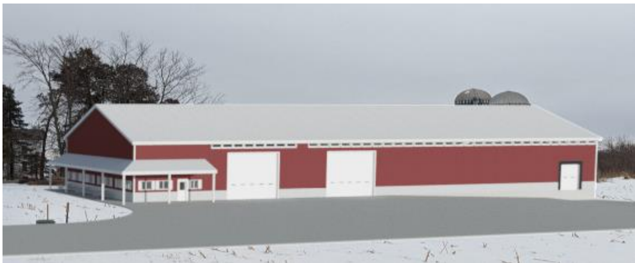
View from Road (entire building)
